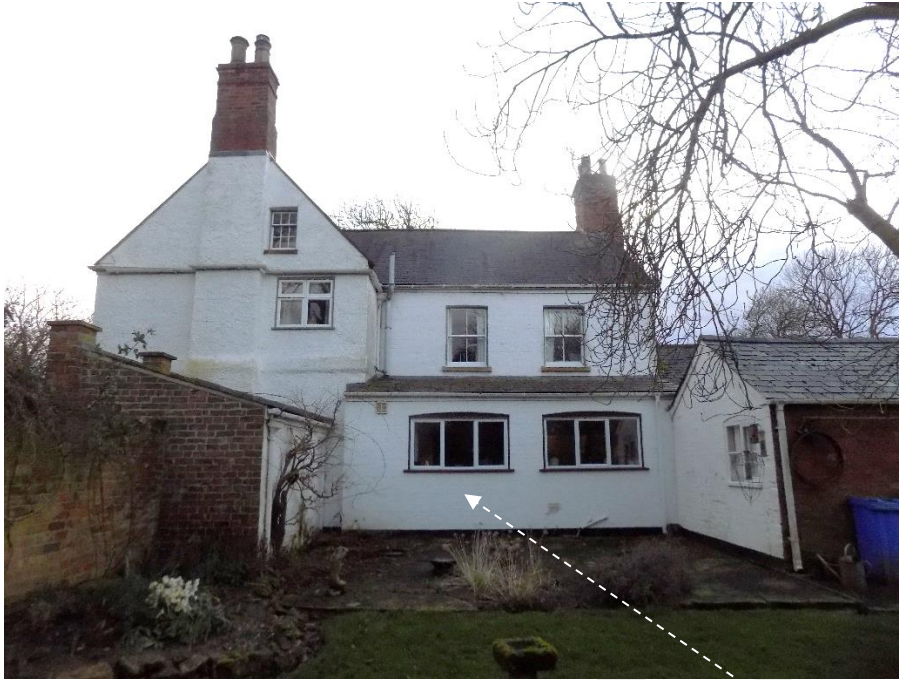
Fig 8, north elevation showing mid-19 th C rear wing, with later 20 th century extension with powder coated metal windows under a segmental brick arch.
