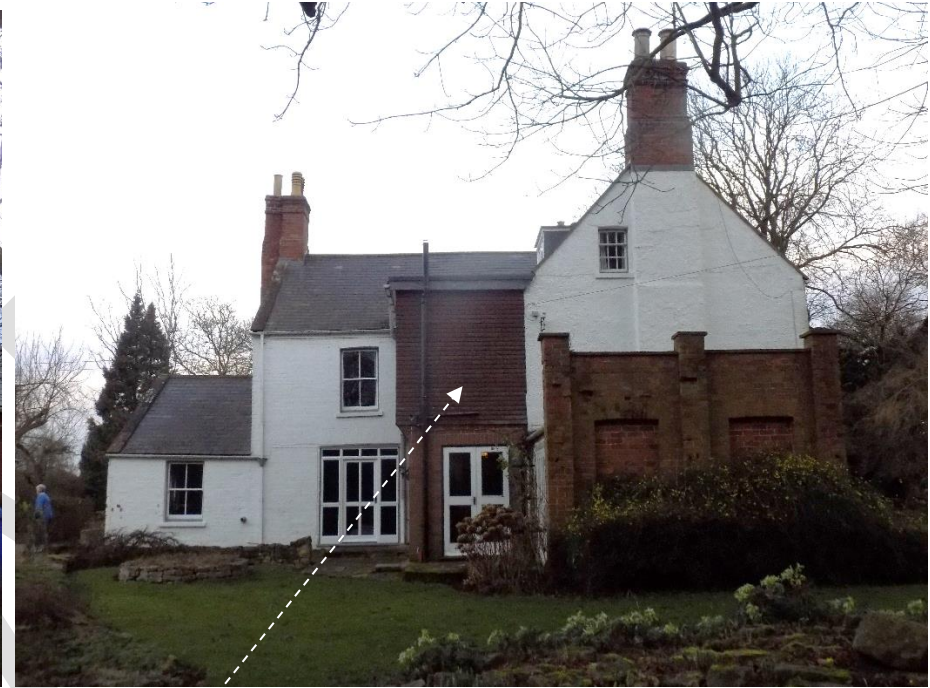
Fig 9, southerly elevation showing mid 19 th single storey addition, the large mid-19 th century rear wing and the circa 1960's flat roofed, yellow brick and timber clad extension.
