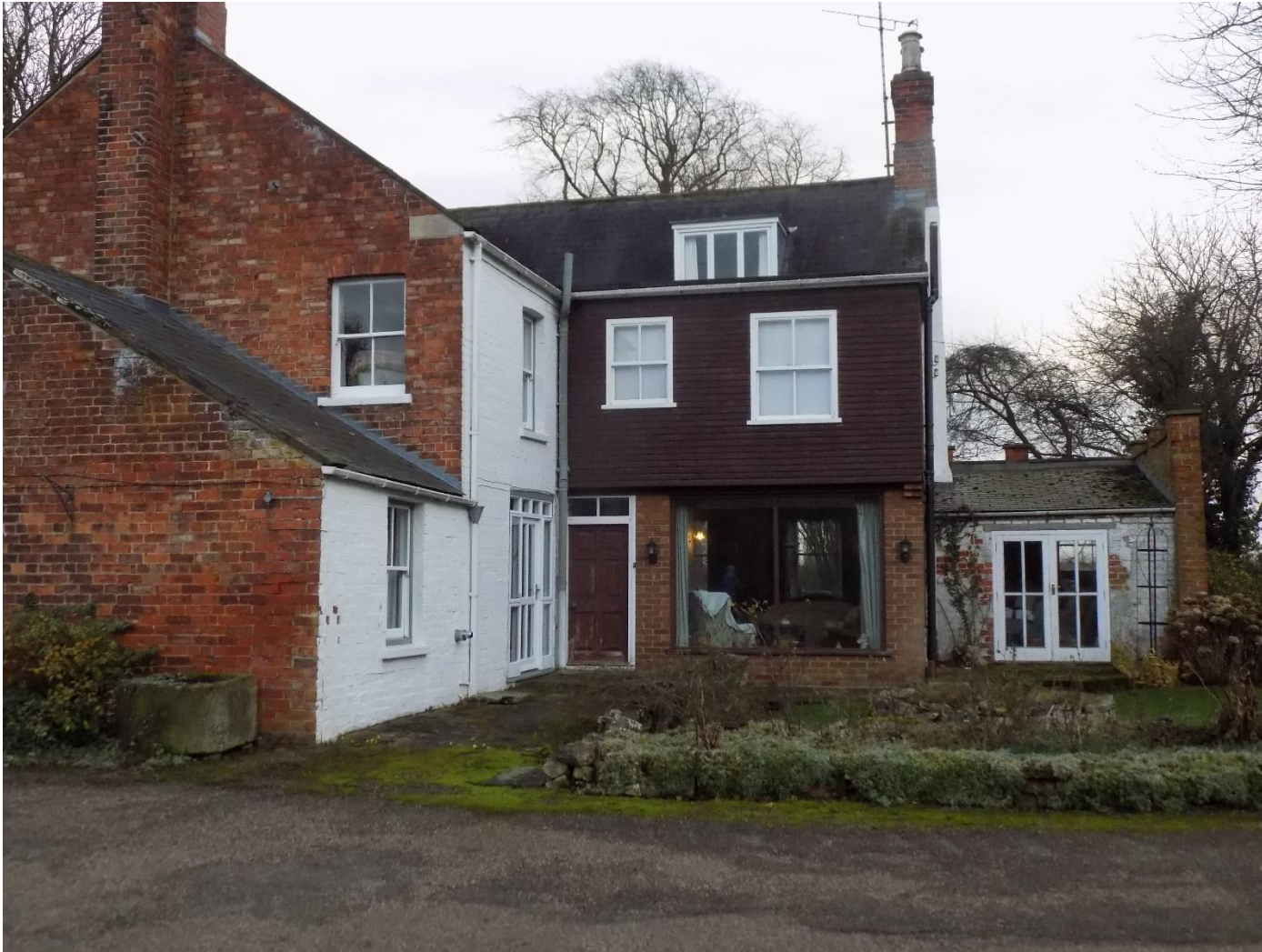
Fig 10, westerly elevation of Burtoft Manor Farmhouse, the 1960's extension with modern six panel door and frame, and a large 'picture' window to the ground floor. Above, timber cladding of circa 1960, and more recently installed vertical sliding sash window. The modern door and picture window are proposed for replacement with a new contemporary aluminium doors. Brickwork and timber cladding will be painted to match the house.
